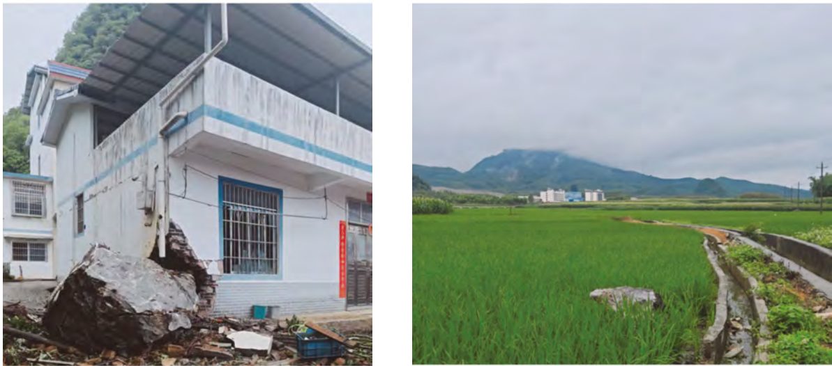
Fig.10 Rockfall triggered by the earthquake in Fengyang Village
