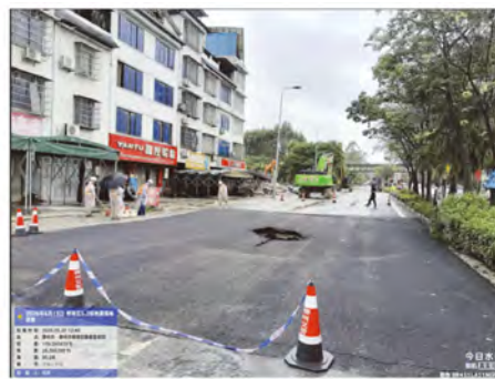
图4 5月18日下午柳太路同一路段发生路面塌陷 Fig.4 Road collapse at the same section of Liutai Road on the afternoon of May 18
