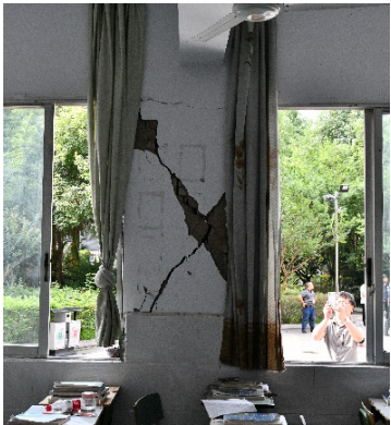
图2 珙一中教学楼花篮梁下的破坏墙段 [1] Fig.2 Damage section of wall in the teaching building of Gongxian Middle School [1]
