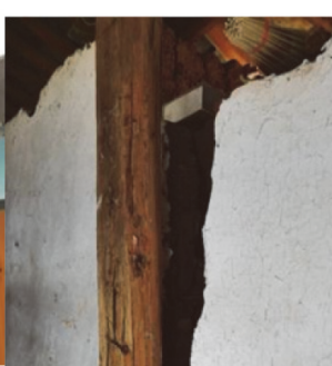
图3 主体架构与墙体分离 Fig.3 Separation of main structure and wall
