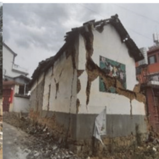
图7 房屋墙体开裂、倾倒 Fig.7 Cracking and toppling of house wall
