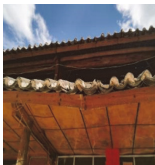
图1 房屋主体出现变形 Fig.1 The deformation of main body of the house
