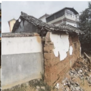
图6 房屋屋顶梭瓦现象 Fig.6 Roof tile phenomenon
