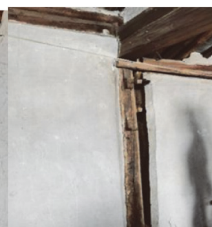
图4 地基沉降造成房屋拉裂 Fig.4 House cracks caused by foundation settlement
