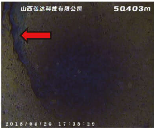
图3 50.403 m处井壁破裂 Fig.3 Fracture of shaft lining at 50.403 m
