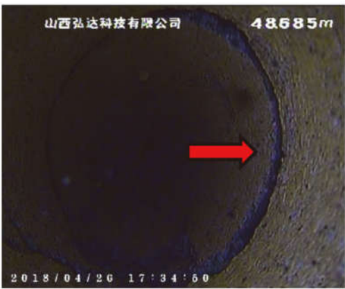
图2 48.685 m处井壁破裂 Fig.2 Fracture of shaft lining at 48.685 m
