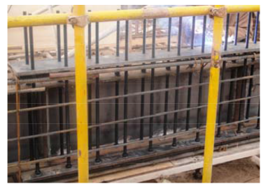
图 2 梁中预埋钢板 Fig.2 Embedded steel plate in beam
