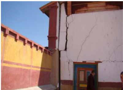
Ⅵ度区墙体轻微裂缝
