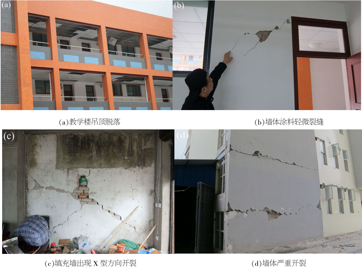
图 1 芦山地震灾区框架结构房屋震害特征 Fig.1 Earthquake damage characteristics of frame structure building in disaster area of Lushan
